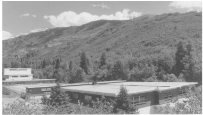
City Creek Water Treatment Plant located about 3 miles above Bonneville Loop Road. Circa 1985
