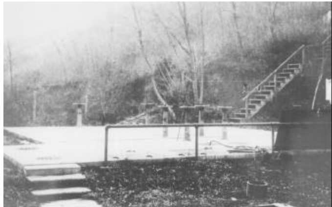
New High Line Intake and 50,000 gallon tank at elevation 5300-ft. The facility was removed in 1953 when the water treatment plant was constructed. Circa 1910.
