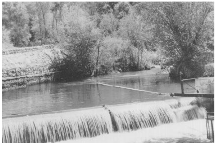
Old High Line Intake (Capitol Intake) above Pleasant Valley Reservoir at the 5058-ft. elevation. Abandoned in 1953 when the water treatment plant was built.
