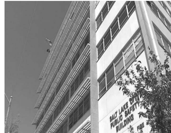
Current Public Safety Building
