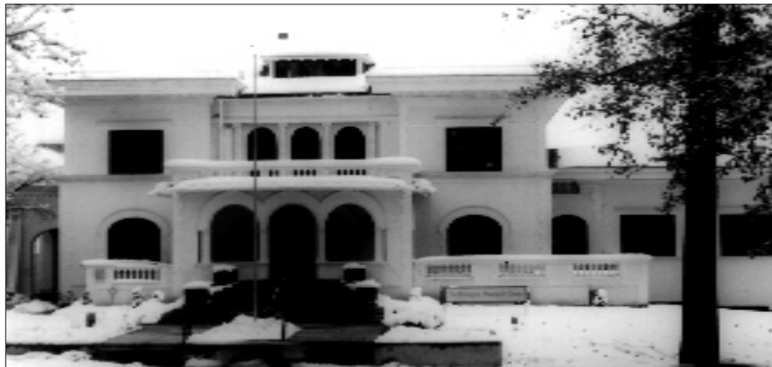
Provide a walkway to the building entry from the public sidewalk.
