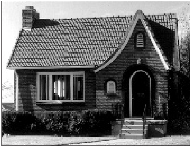
This bar-tile replacement roof would be more appropriate for a Spanish Colonial Revival style building. In the case of a Tudor Revival structure as shown above, the bar-tile roof is overpowering and is inconsistent with roof materials historically used for this style.
