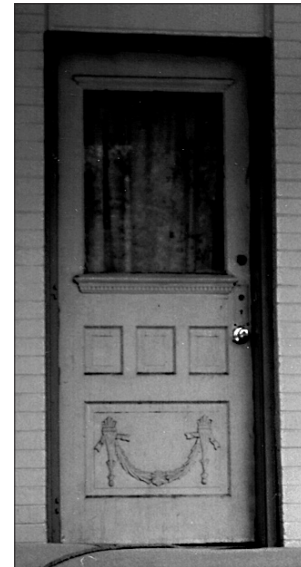
The original materials and details of a door contribute to the overall historic character of a building and should be preserved.
