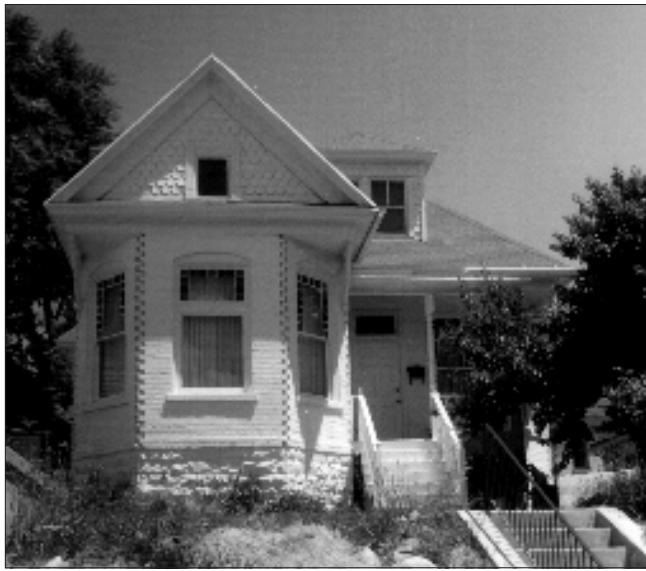
Decorative shingles in the gable, turned posts on the porch and the interlocking brick bay of this house exhibit the high degree of craftsmanship and attention to detail that mark many houses in the neighborhood.
