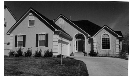
This Avenues house was constructed in 1993. The builders rotated the garage so that the doors would not be a dominating streetscape feature, thus maintaining the traditional "pedestrian-friendly" quality of the street.
