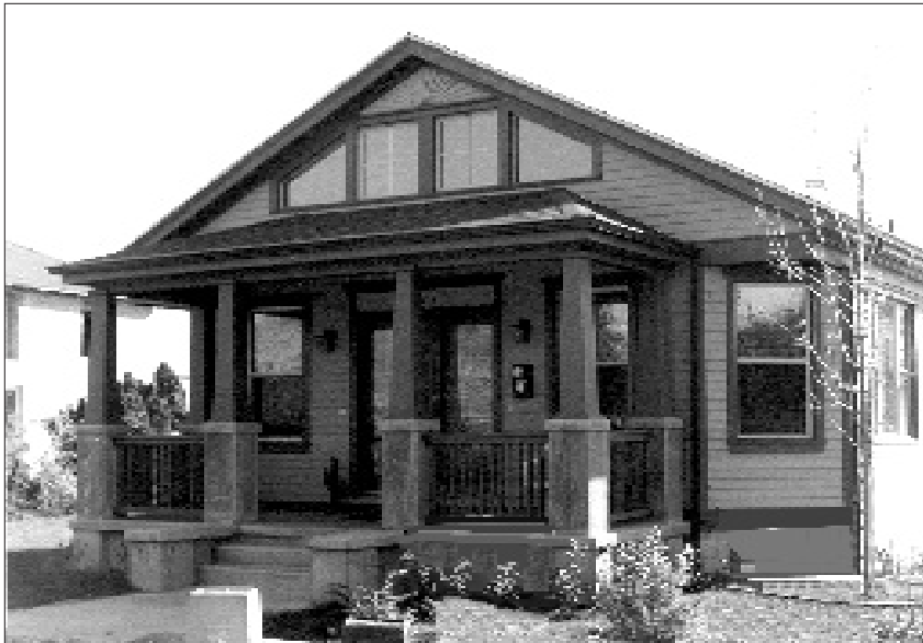
Windows and doors should be framed in materials that appear similar in scale, proportion and character to those used traditionally in the neighborhood.
