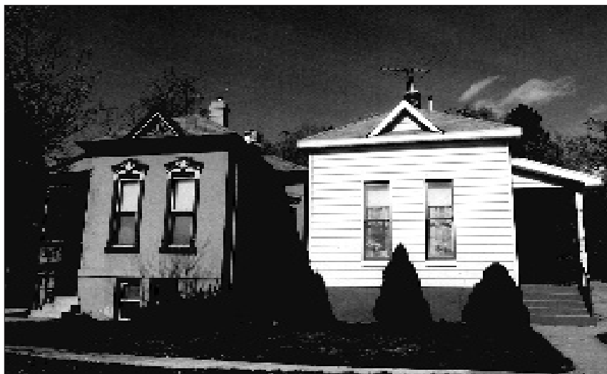
The house on the right is clad with siding that obscures the original material, which is similar to that of the house on the left. Such coverings are not allowed in historic districts.
