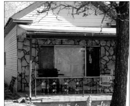
Covering original building materials with new materials is not allowed. This rock veneer, for example, obscures the original wood siding.
