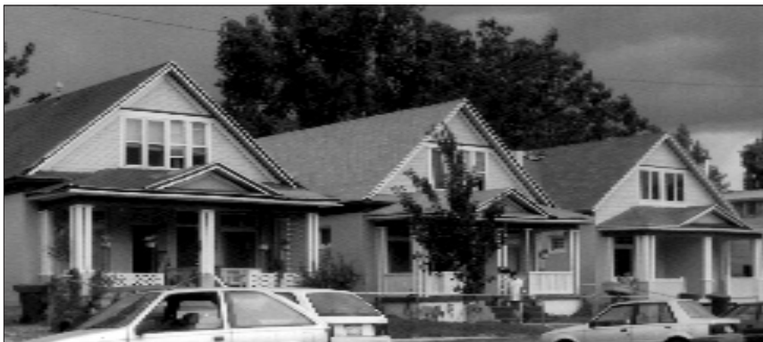
The uniform setback of these vernacular structures provides a sense of alignment and the porches provide a consistent orientation to the street.
