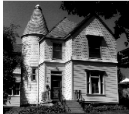
A two story frame structure of the Victorian era. The porch has been altered.
