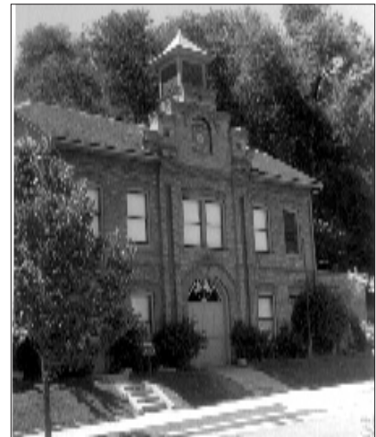
Ottinger Hall was constructed in 1900 for the Volunteer Firemen's Association.
