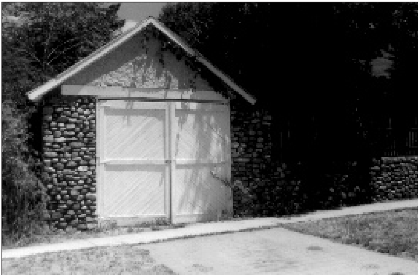
When treating a historic accessory building, respect its character-defining features such as primary materials, roof materials, roof form, historic windows, historic doors and architectural details.
